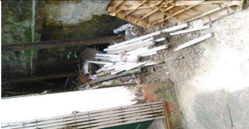
Exhibit 1 - Improper damaged tube light storage facility
