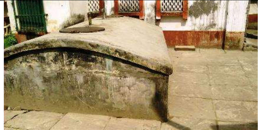
Covered underwater storage tank
